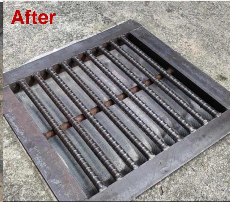
Install aluminium screen as drain filter to prevent resin flow into drain
