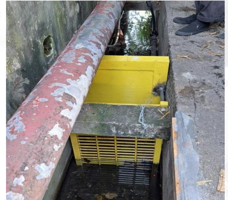
Install resin grease trap at end outlet of drainage
